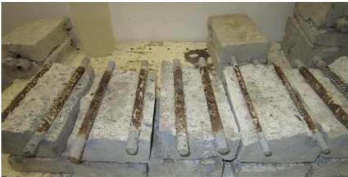
Fig 2 Photograph of split reinforced concrete prisms showing the corroding reinforcements
